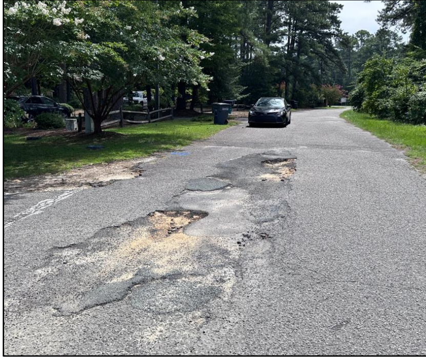
Figure 6: Dover Street Existing Conditions
