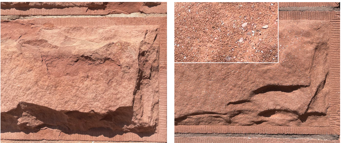
Figure 13. Cast stone was used to effectively replace individual blocks of sandstone. Both the original (left) and the substitute material (right) retain similar physical and visible properties. Having weathered for over 30 years, some erosion of the binder has revealed quartz grains of the aggregate (inset), but it is only noticeable upon close inspection. Photo: John Sandor, NPS.
