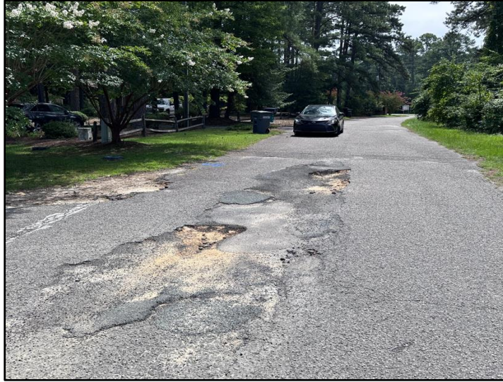
Figure 7: Dover Street Existing Conditions
