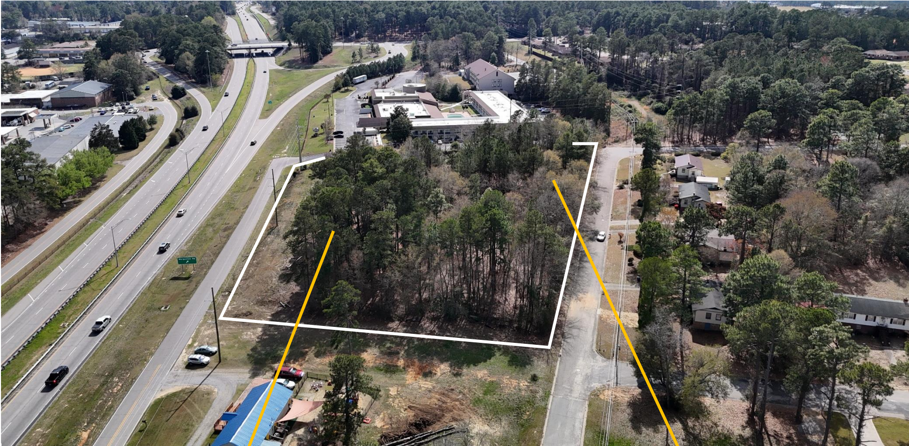
Figure 1. Drone Imagery of the Subject Parcels (Facing South)
