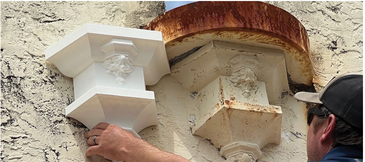
Figure 23. 3-D printing using various polymers is occasionally used to replicate missing metal or wood features. This new application is continually being refined, but the application can be successful when a painted, lightweight feature needs to be replicated. Photo: NPS.
