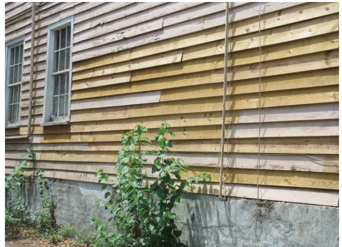
Figure 3: Incremental repair is best done using in-kind material to minimize differences in the performance characteristics that could negatively affect the overall assembly. Photo: NPS.
