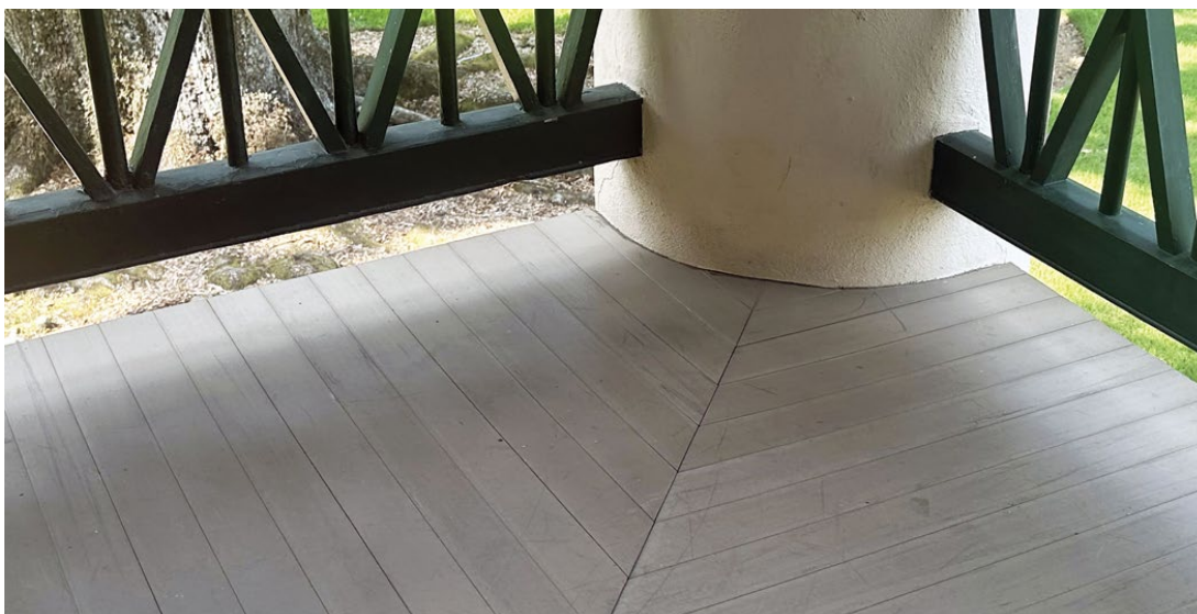
Figure 15. Tongue-and-groove porch flooring is manufactured in several different substitute materials. Each type has different properties, though most are more moisture-resistant than wood. The prefinished product shown can be painted when worn, but repainting is not recommended for some product choices. Photo: Oak Alley Foundation.
