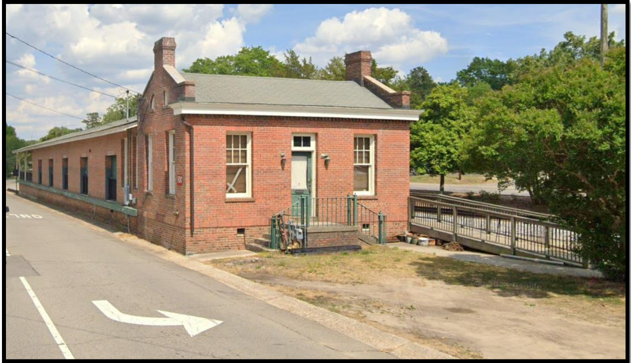
305 NW Broad Street – “South-West Façade.” Google Maps, retrieved June 30, 2025.
