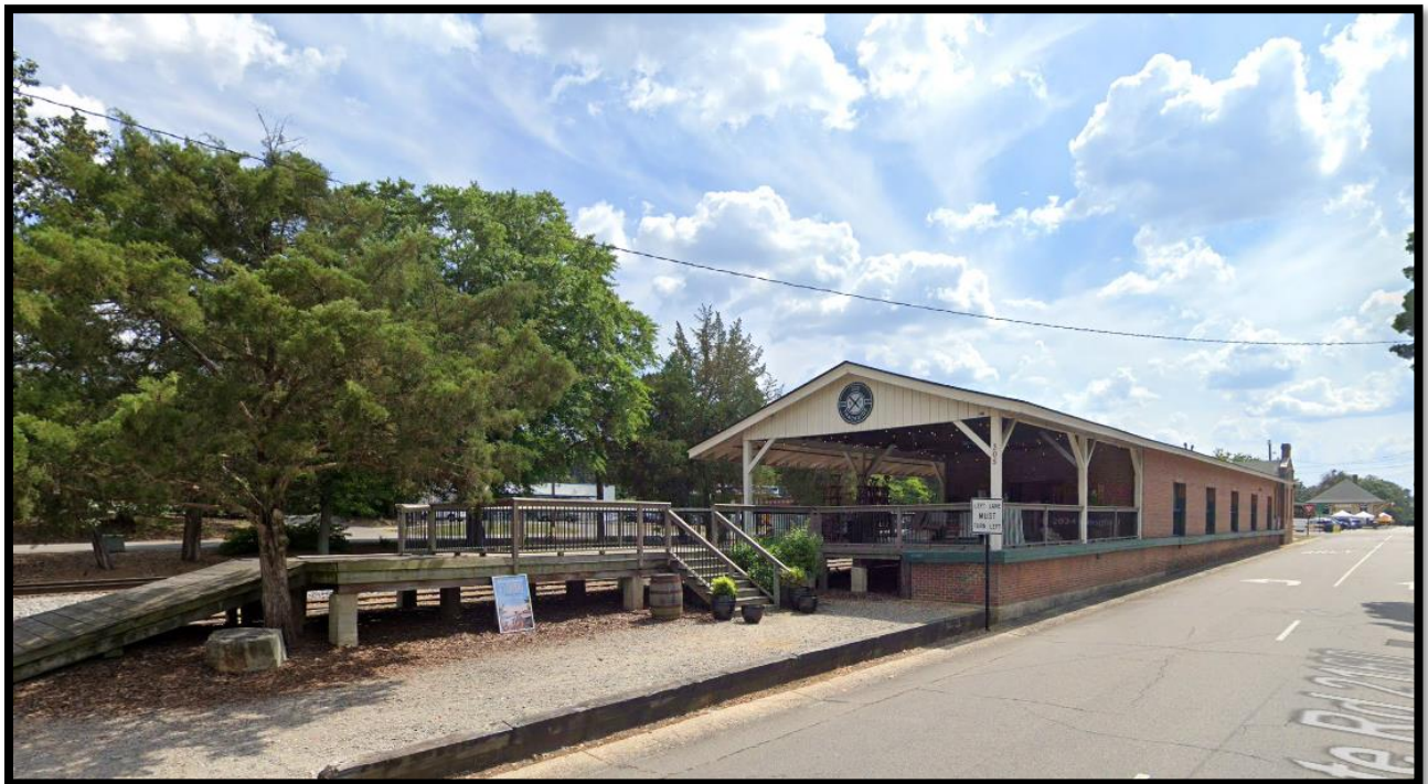
305 NW Broad Street – “North-East Façade.” Google Maps, retrieved June 30, 2025.
