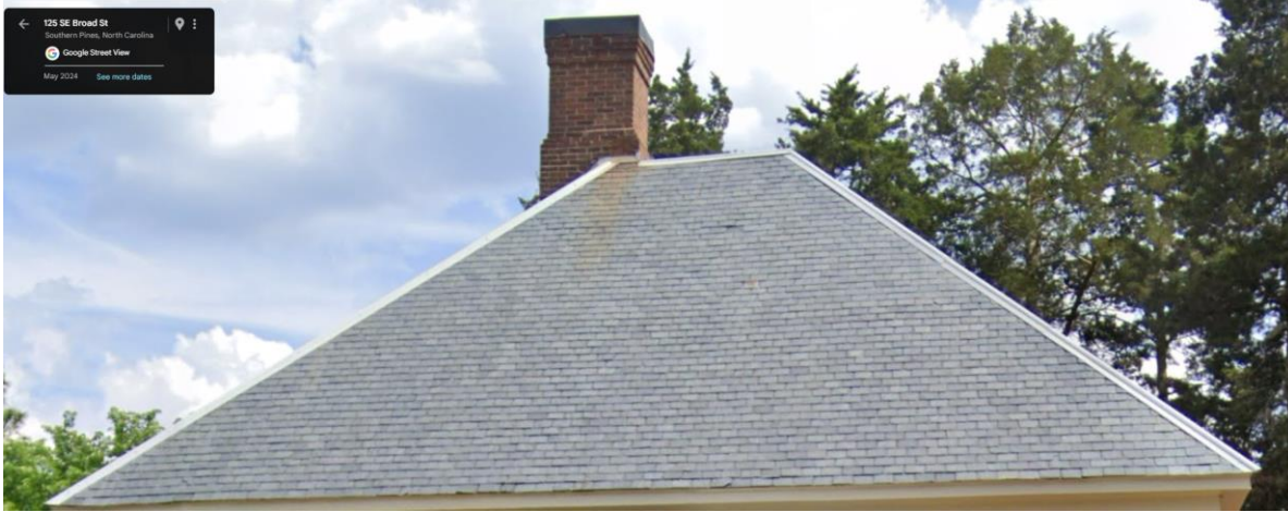
Figure 4: Ridge caps as seen from Broad Street. (Photo provided by staff)
