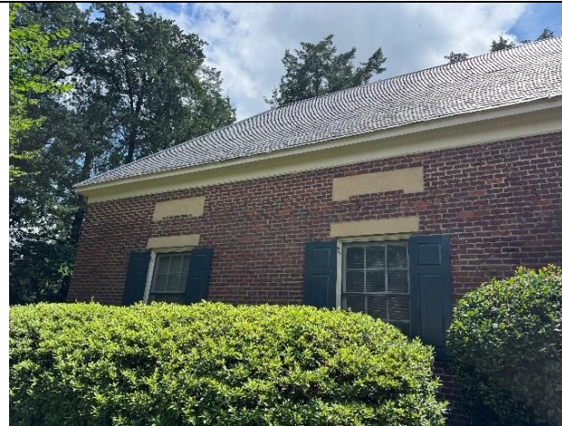
Figure 5: Pennsylvania Avenue-facing elevation, displaying a lack of drip-edges. (Photo provided by staff)
