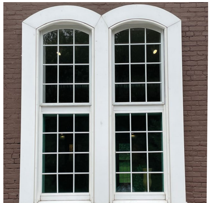
Figure 9. Previously bricked-in openings below the flood line were reopened and new aluminum windows installed with cellular PVC trim detailed to hold back moderate flood waters and survive exposure to water. Photo: John Sandor, NPS.
