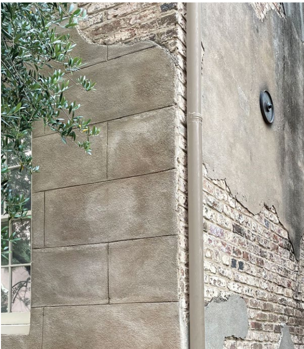
Figure 2c. Stucco has been used to imitate a number of building materials for many centuries. Seen here, stucco was applied to a brick structure and scored to represent a stone façade. Photo: John Sandor, NPS.
