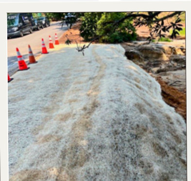
Hunter Trail Repairs
