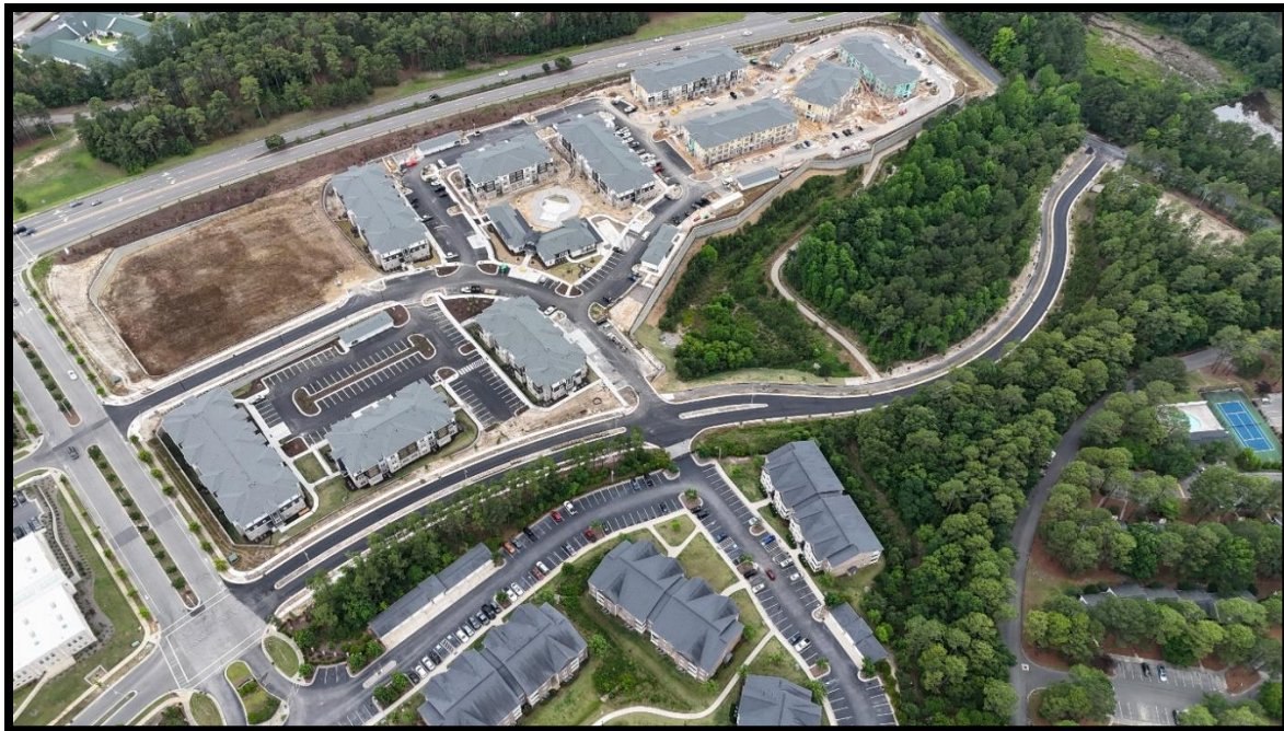
Figure 2: Aerial Photo of Air Tool Drive (Taken May 30, 2025)
