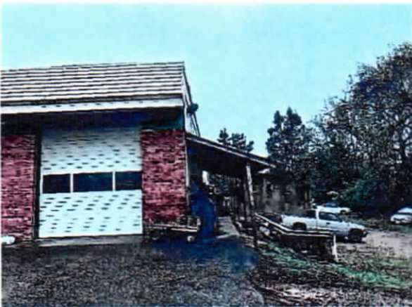
View of side and back of subject exterior of front building.
