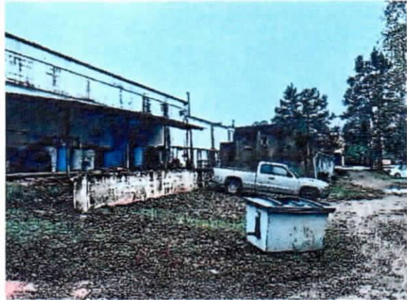
View of back of front building and side of back building.
