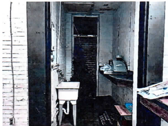
Garage wash area.
