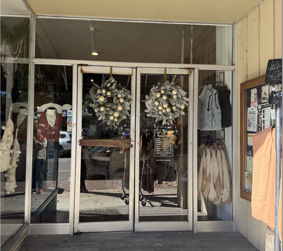
Existing Doors (Metal and Glass)
