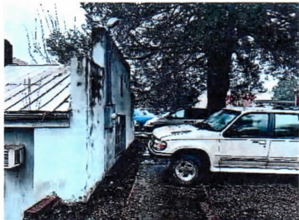
View of side of back building.
