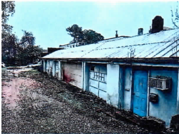
View of back building.
