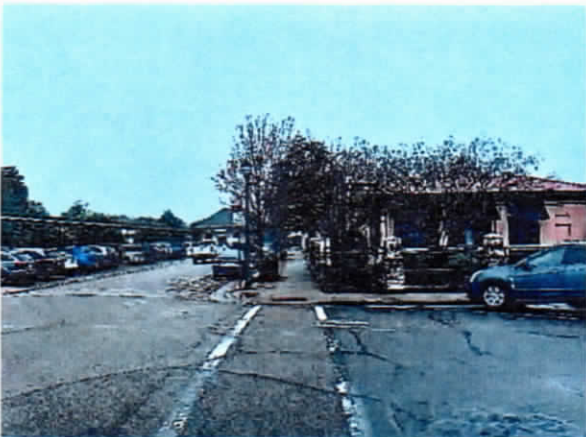
Street view of front building towards retail shops.
