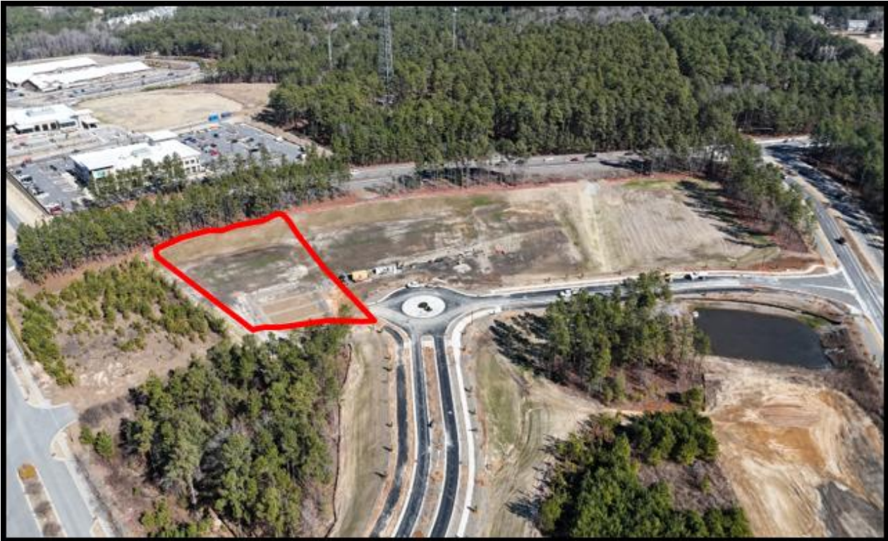
Figure 1: Vicinity Arial Image Conditions
