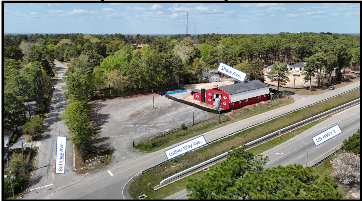
Figure 3: Drone overhead facing N. West
