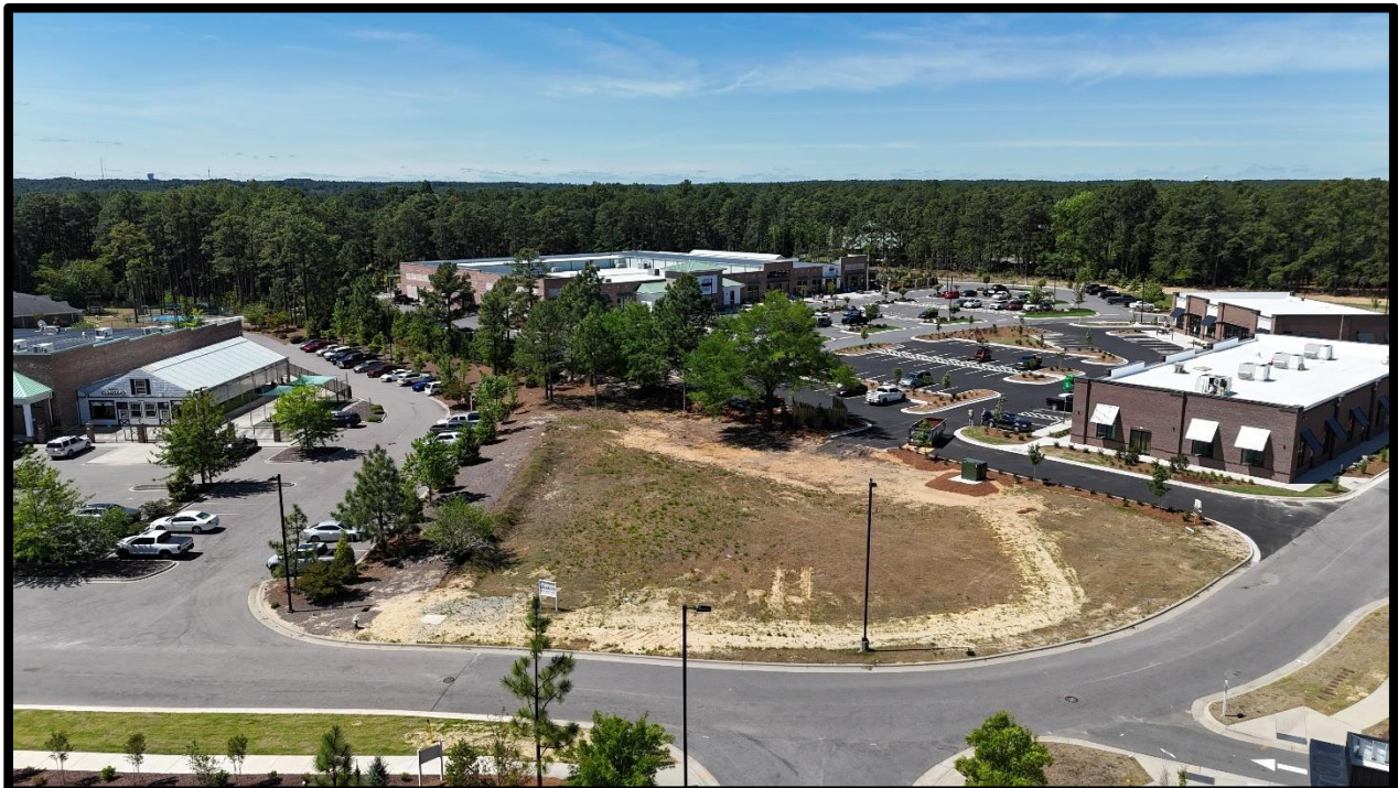
Figure I: Vicinity Arial Image Conditions
