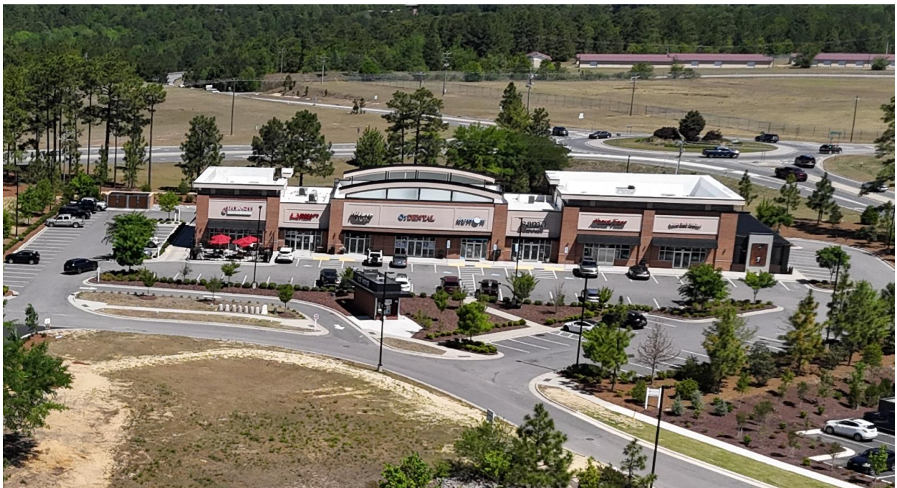
Figure 4: Original Commercial Building at Tyler's Ridge
