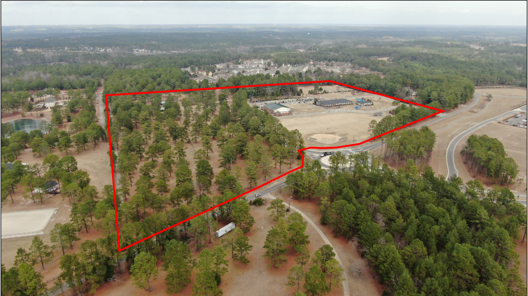
Figure 2: Aerial Image Looking Northeast at Subject Property (February 25, 2022):
