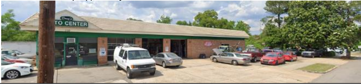
Figure 3: Existing Conditions viewed from W. Connecticut Avenue
