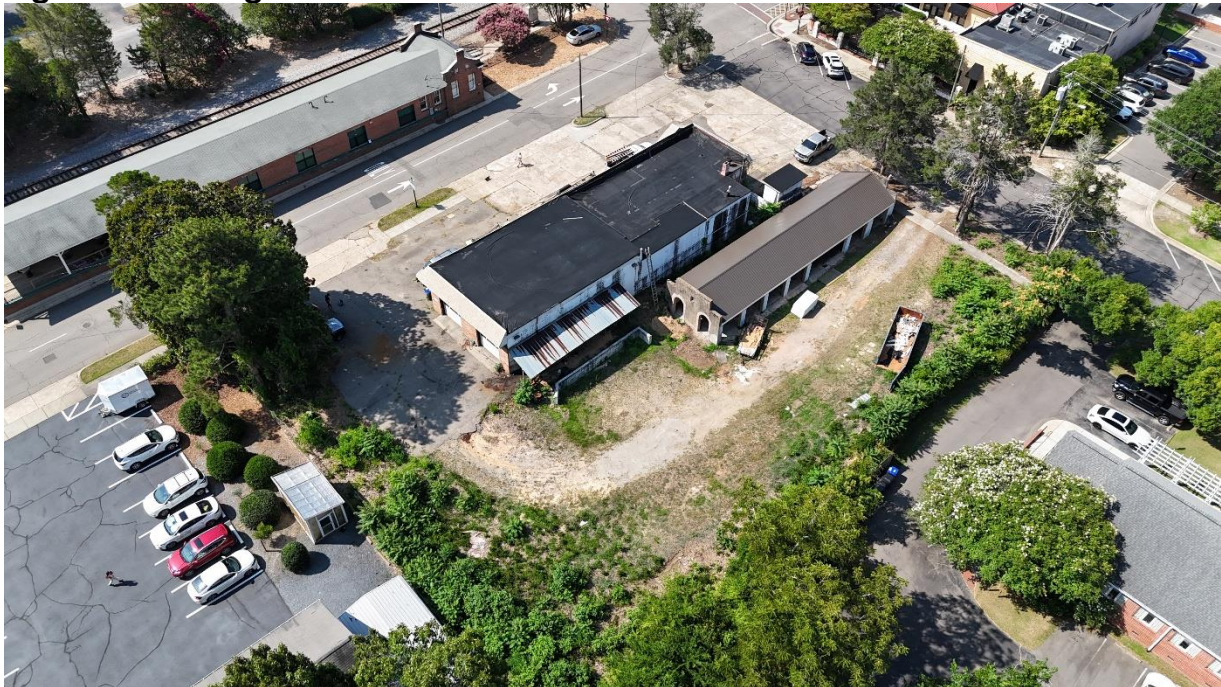
Figure 4: Existing Green House Aerial
