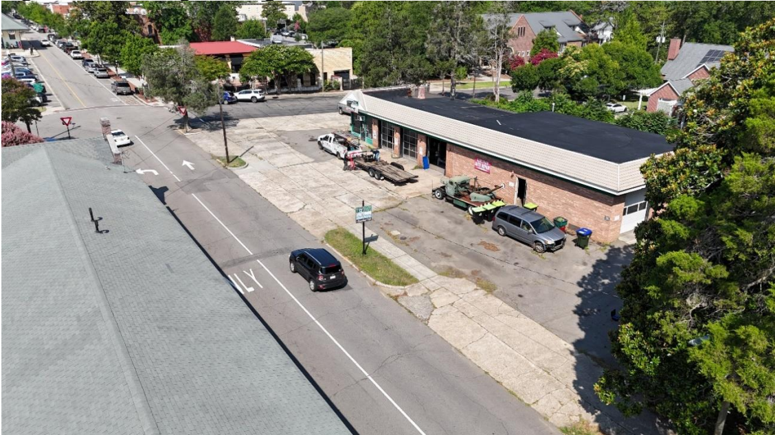
Figure 18: Existing Parking Conditions, Viewed from NW Broad
