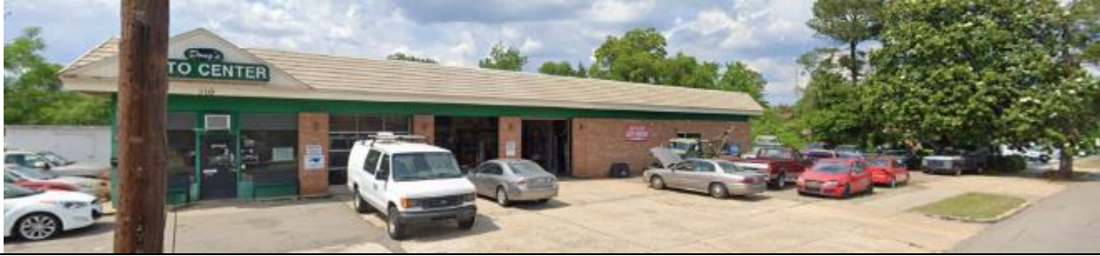
Figure 3: Existing Conditions viewed from W. Connecticut Avenue
