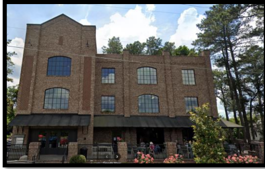
Figure 10: Mews Building at 280 NW Broad Street (Adjacent to subject property) comprised of stucco.
