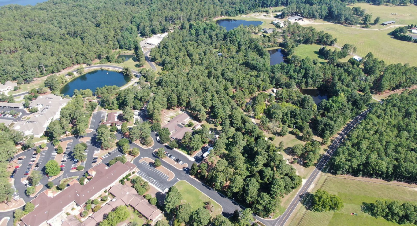
Figure 2: Aerial (Drone) Image of Present Condition of Subject Property (August 4, 2022):
