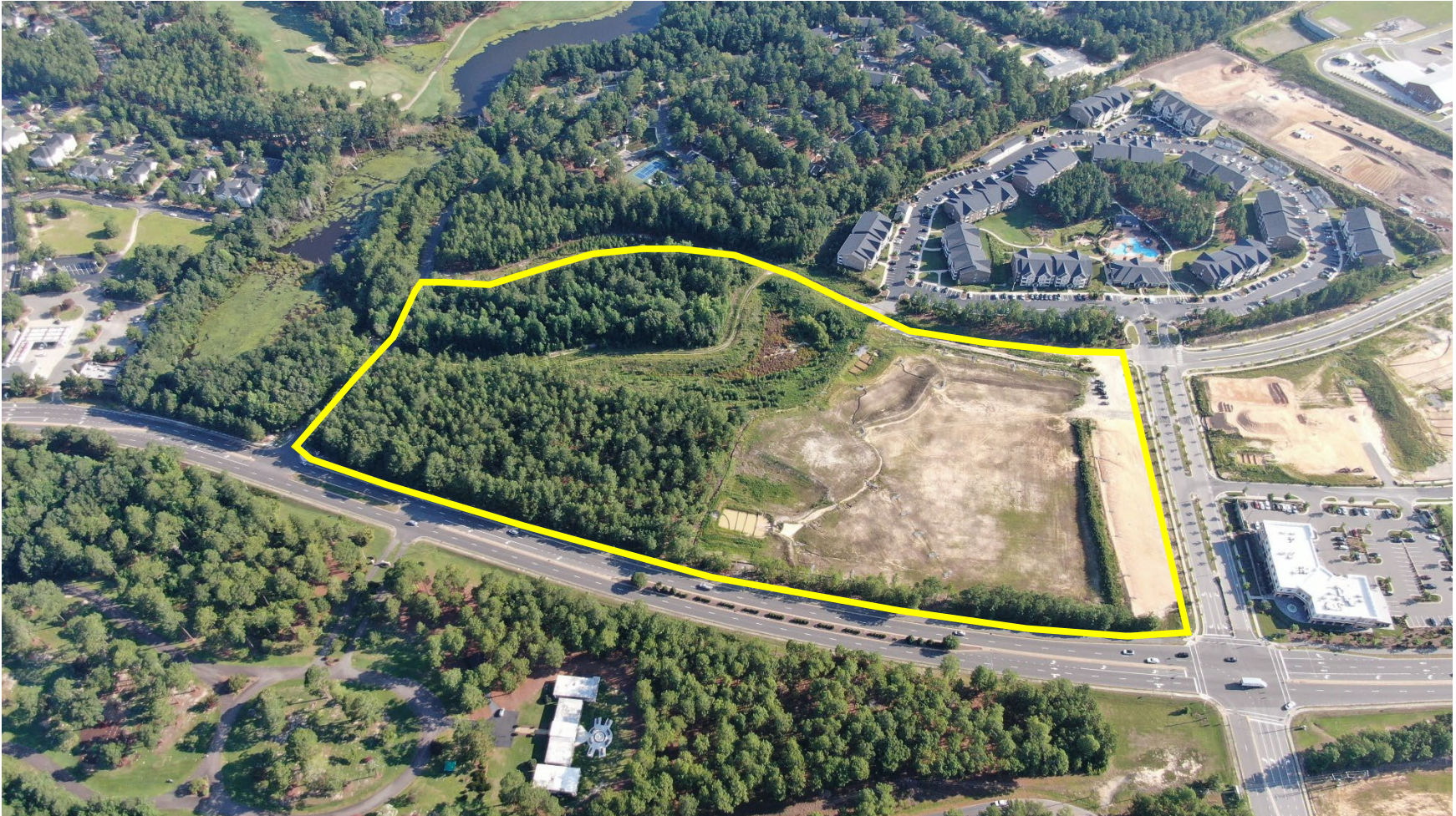
Figure 1: Aerial image taken over the site, looking north towards Legends Apartments and Mid South (approximate location of current phase shown in yellow)
