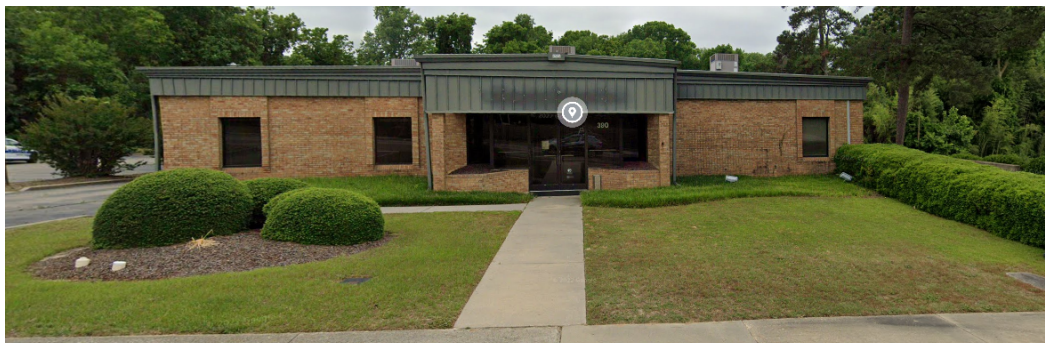
Existing Front Elevation Image
