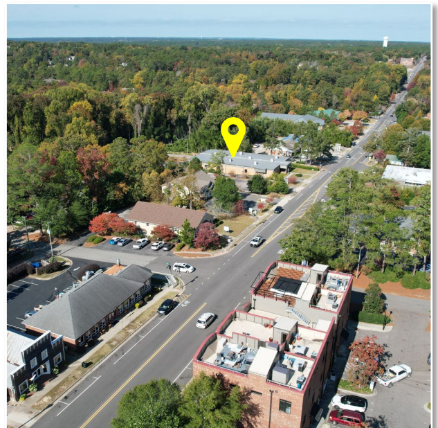
Drone-Captured Image of Subject Property Looking Northwest on W. Pennsylvania Ave. as of October 28, 2022.
