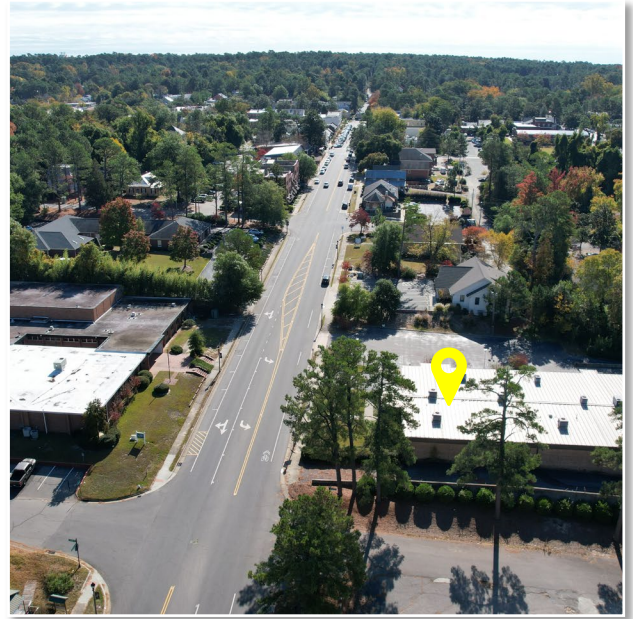
Drone-Captured Image of Subject Property Looking Southeast on W. Pennsylvania Ave. as of October 28, 2022.
