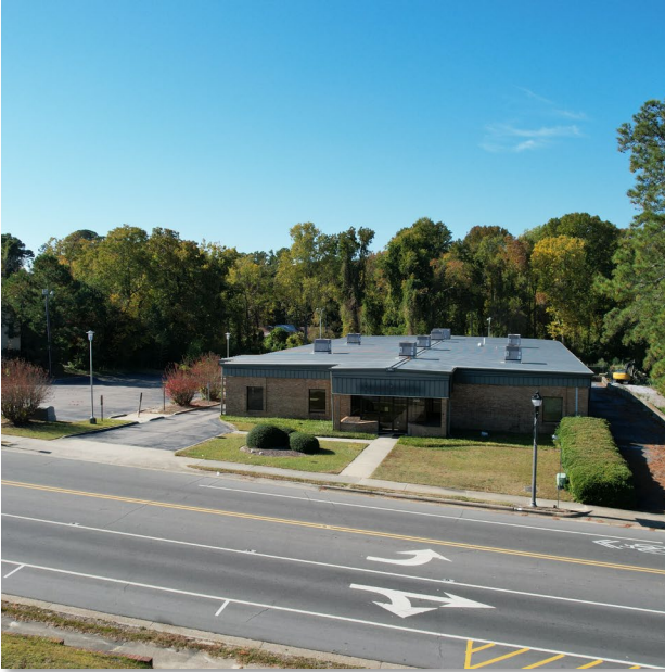
Drone-Captured Image of the Front Elevation of the Existing Building and Side Yards as of October 28, 2022.
