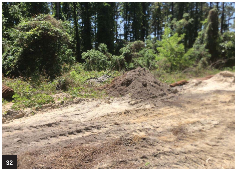
Topsoil pile in materials storage area located in the east-central portion of Area 2
