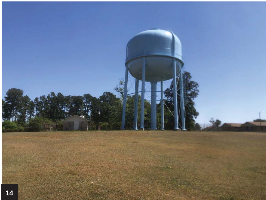
Water tower in northern portion of Area 1
