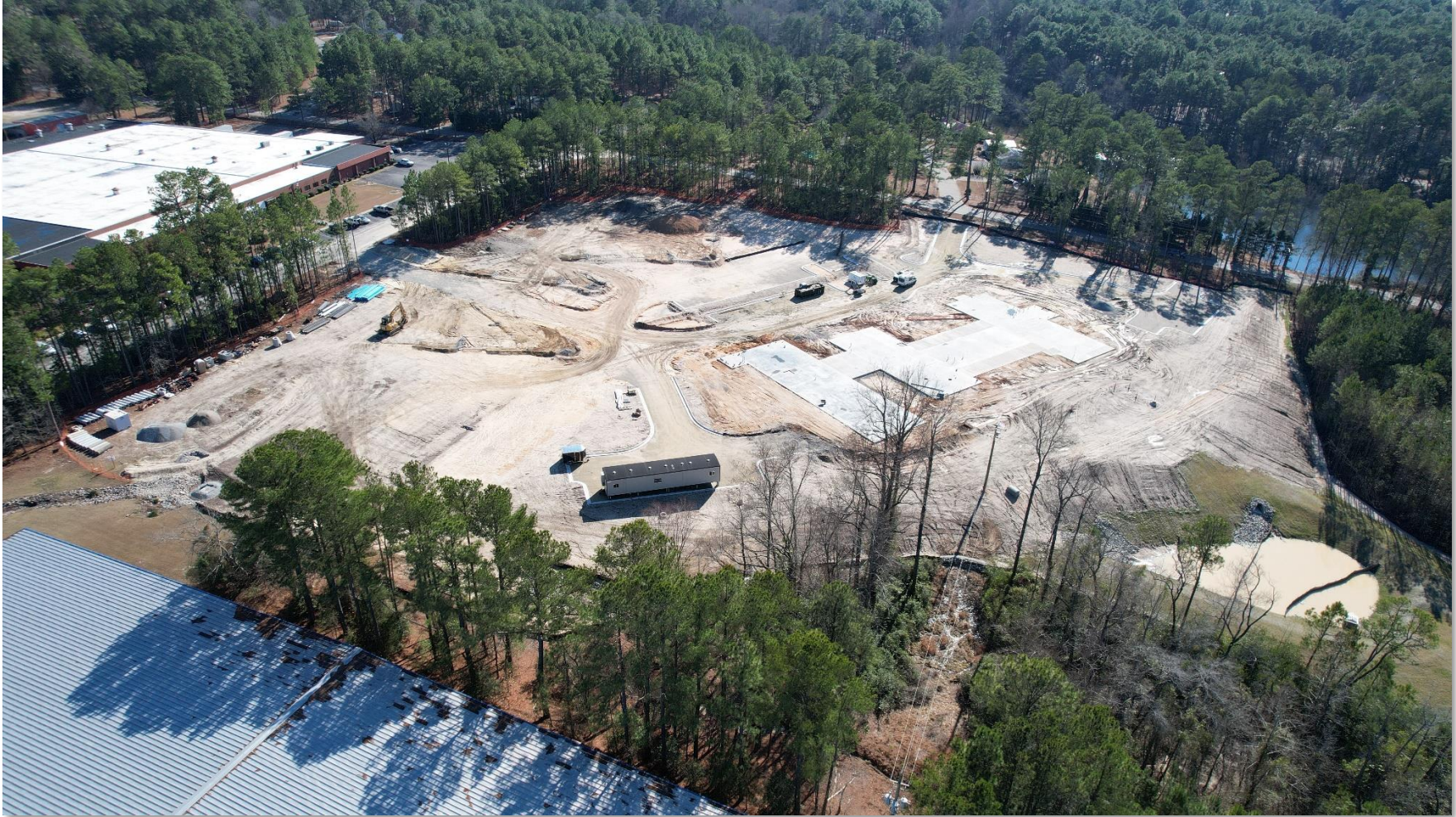
Figure 5. Drone footage of on-going construction on the subject property, looking southeast (February 3, 2023).
