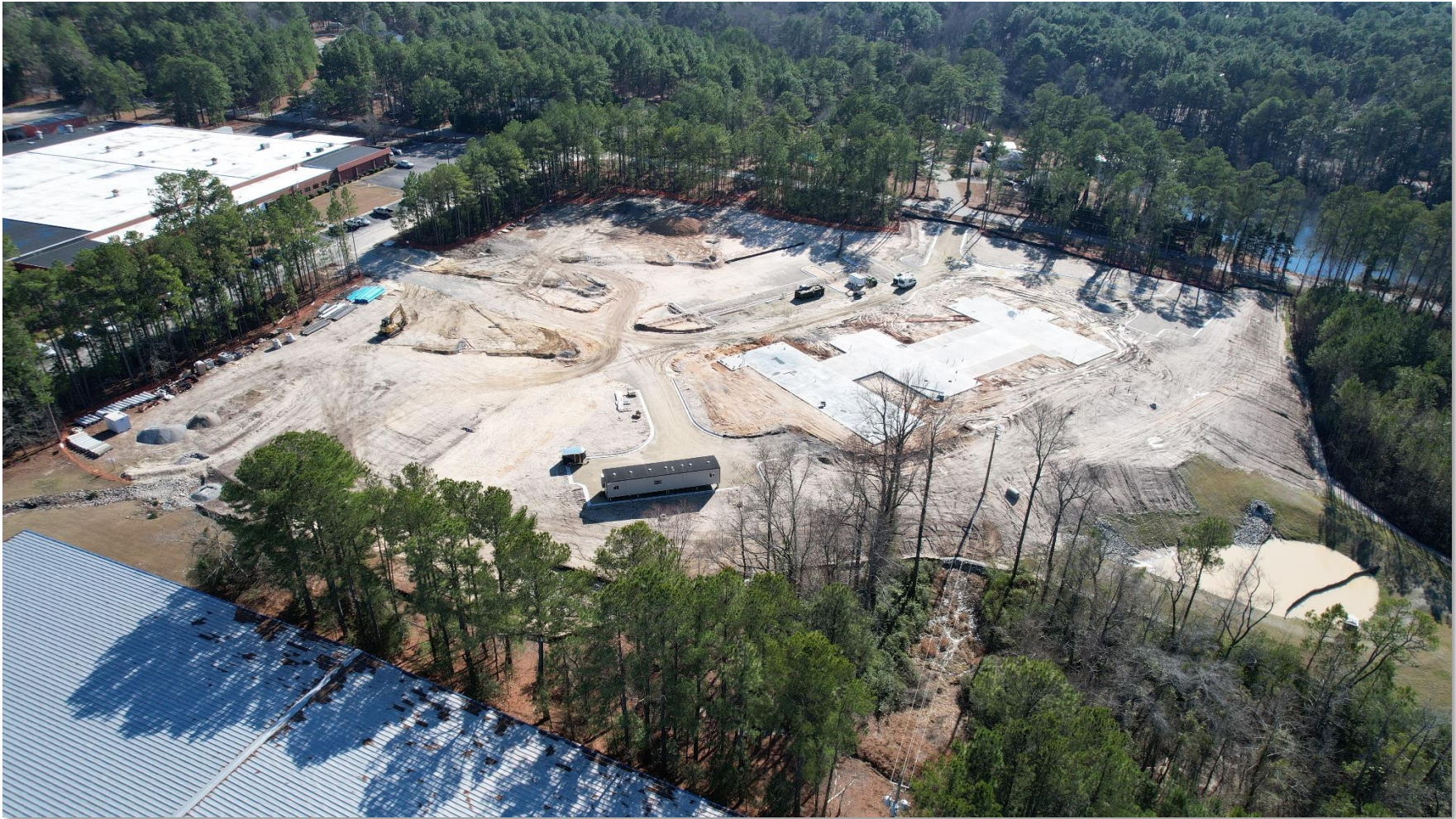
Figure 5. Drone footage of on-going construction on the subject property, looking southeast (February 3, 2023).
