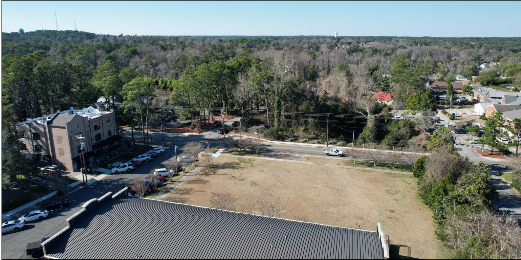
Figure 3: Oblique Aerial Image of Present Condition of Subject Property (February 3, 2023):
