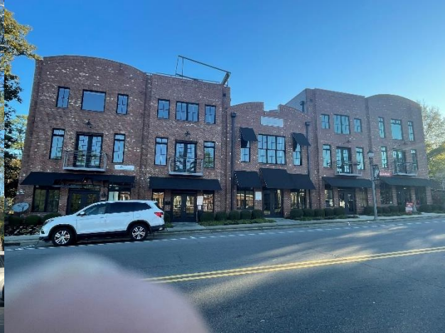
The Pinnacle Building (note the loft on unit 2)
