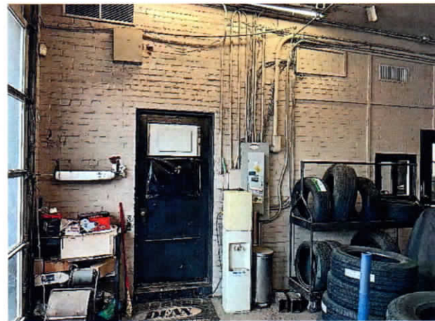
Garage entrance to reception area.
