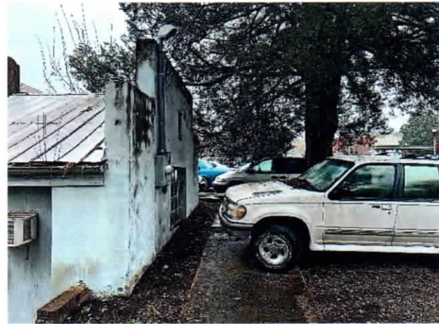
View of side of back building.
