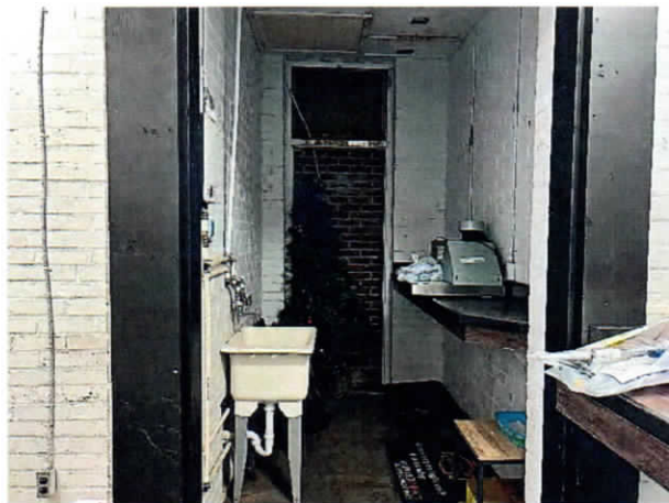
Garage wash area.
