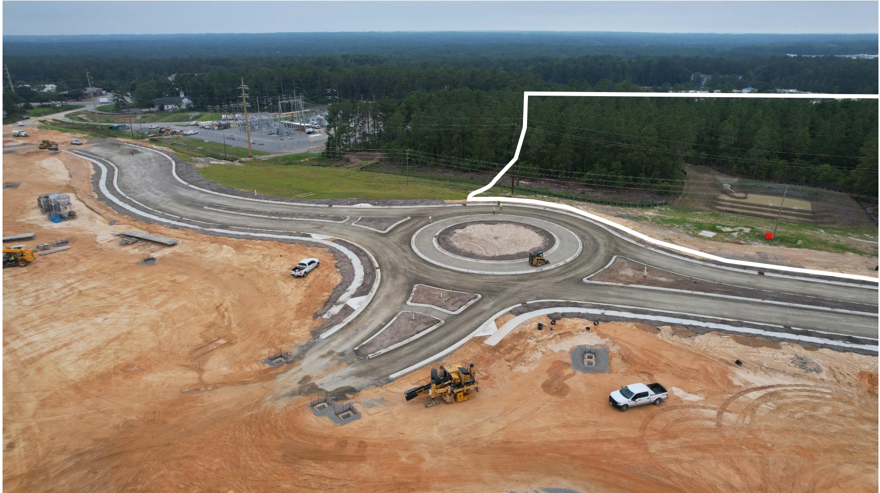
Figure 3: Drone image taken July 13, 2023, showing Carolina Green Parkway Roundabout Construction.
