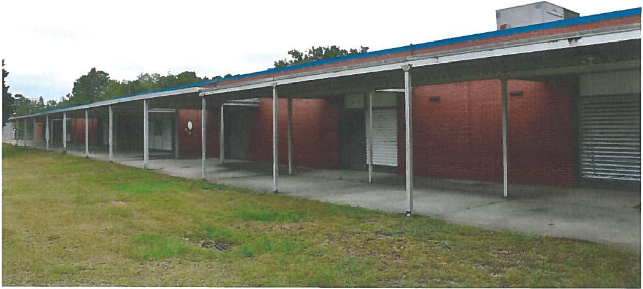
1978/1988 Classroom building, south elevation, looking west.
