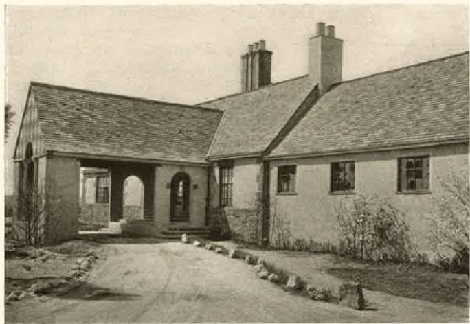
Detail of Entrance Front
