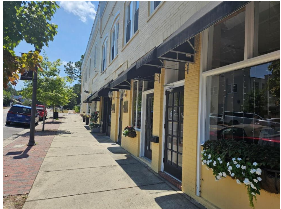
Existing awnings on Pennsylvania Avenue side of building (110-122 W Pennsylvania)
