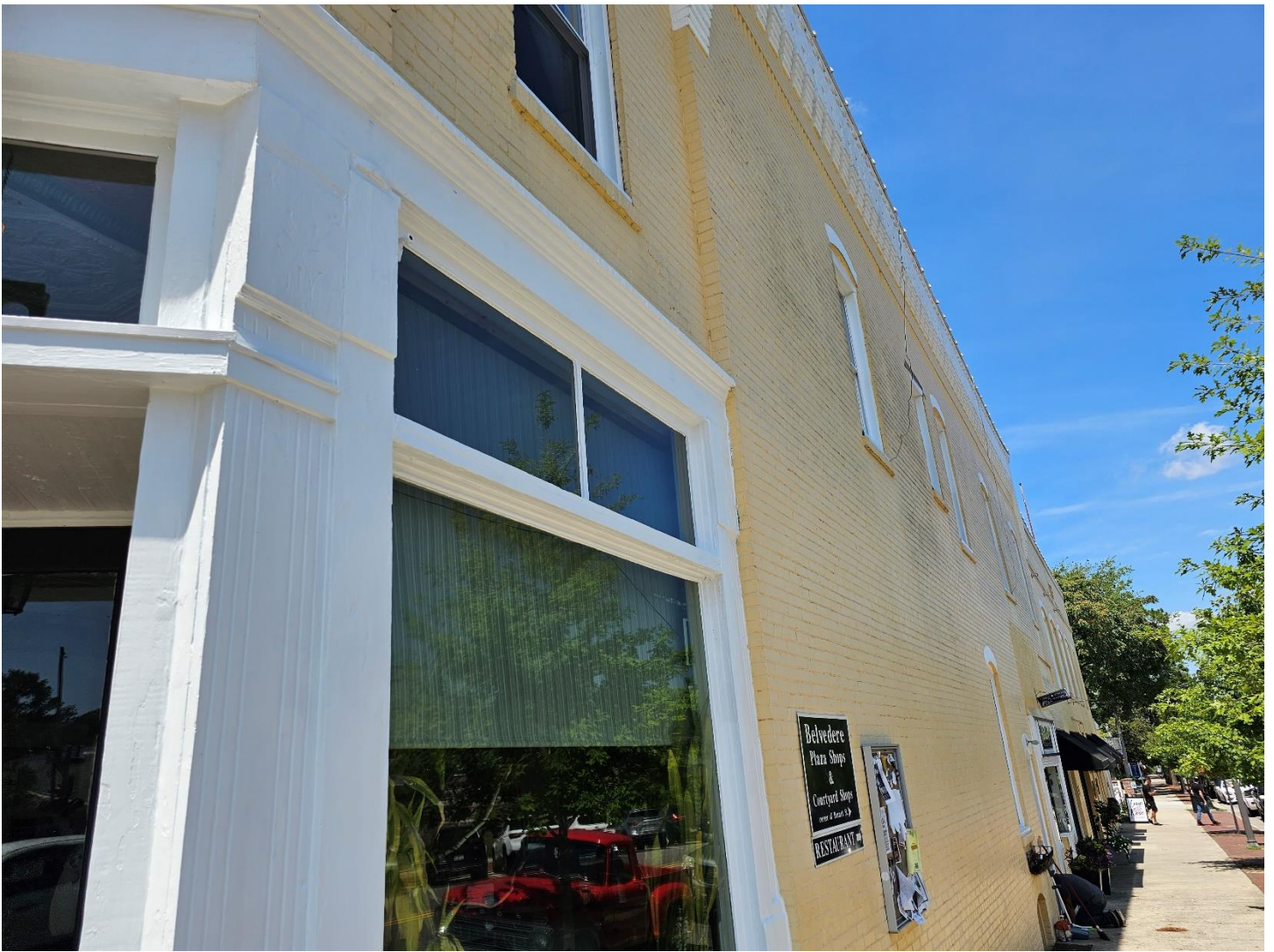
Proposed site for 8' black awning, 125 SW Broad Street (facing Pennsylvania Ave)
