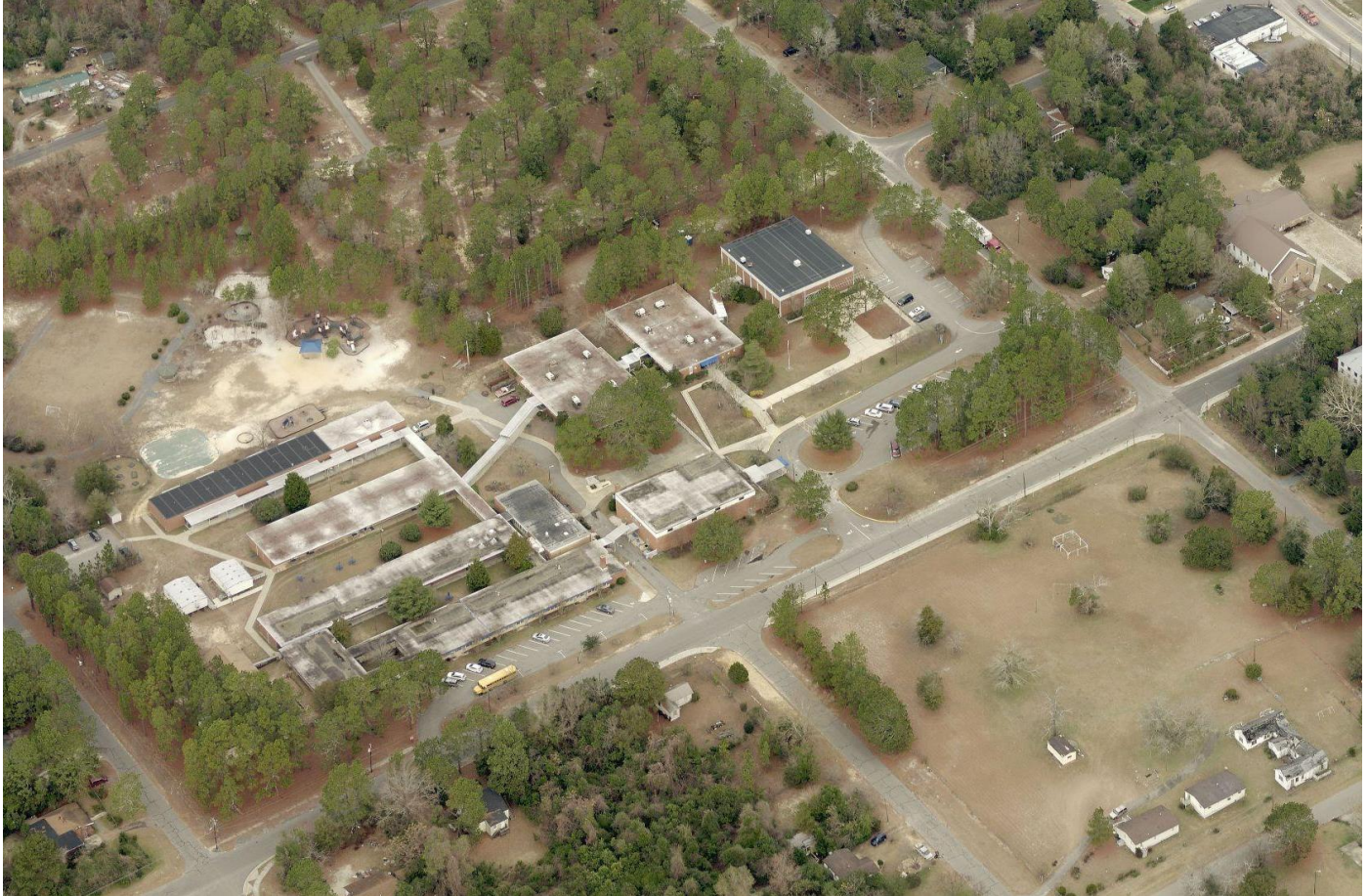
Figure 1: Aerial view of the property
