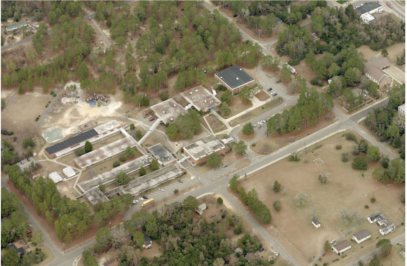
Figure 1: Aerial view of the property
