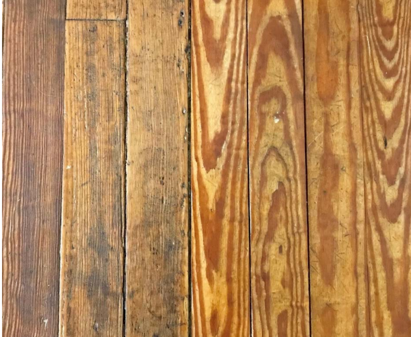
Fig. 1. 90-year-old tight-grain yellow pine quarter-sawn flooring to the left and flat-sawn yellow pine patch to the right. While flat-sawn lumber was commonly used for flooring, quarter-sawn lumber is more expensive due to the method of cutting a log into four quarters followed by plain sawing each quarter. There is also more waste material with this method but the result is a lumber that is more stable (absorbs less moisture with the tighter grain and grain orientation) and less likely to cup and warp. Older flat-sawn and quarter-sawn flooring typically contains more heartwood and less sapwood than today's lumber.
