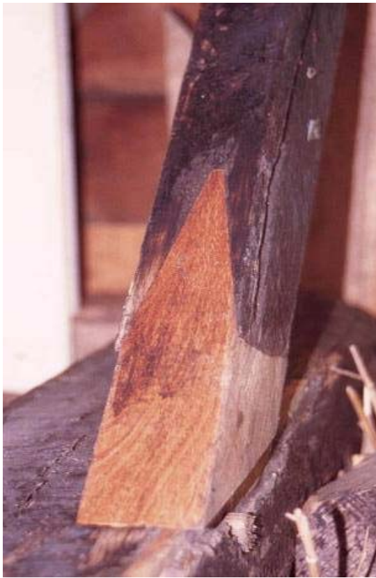
Fig. 5. Traditional "Dutchman" repair
