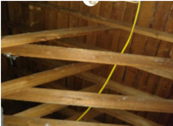
8.2 Wood trusses in the attic
