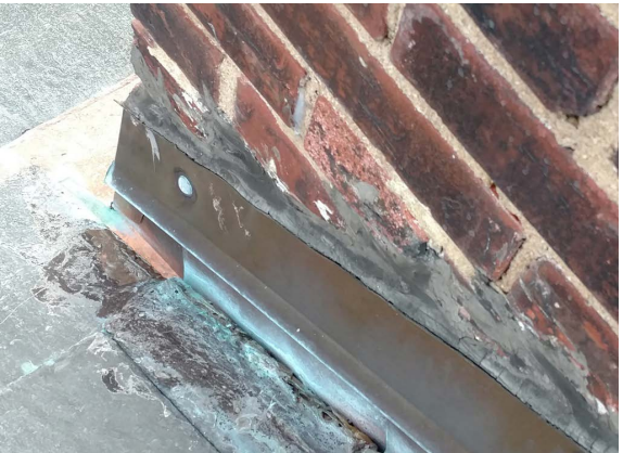
4.8 Chimney flashing
