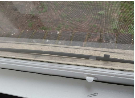
3.2 Typical interior view of the windows
