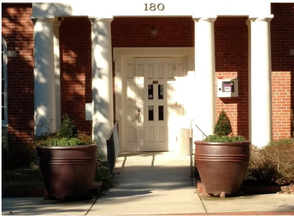
2.1 Main entrance door
