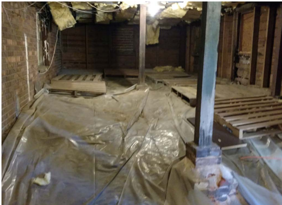
8.1 Brick walls and interior wood columns
