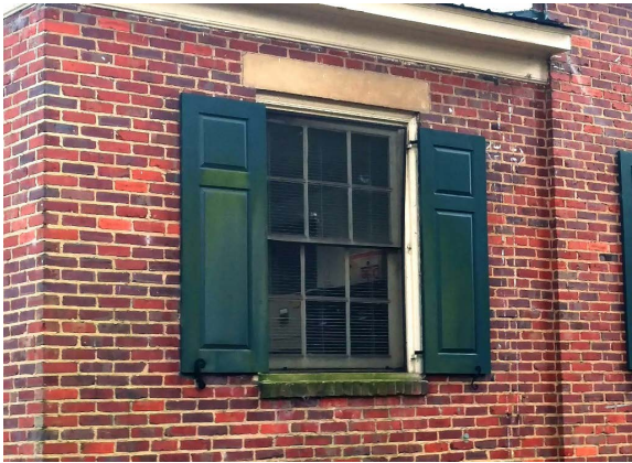
3.1 Typical exterior window
