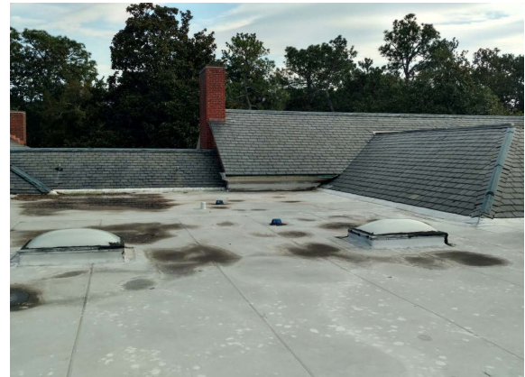
4.1 General roof overview
